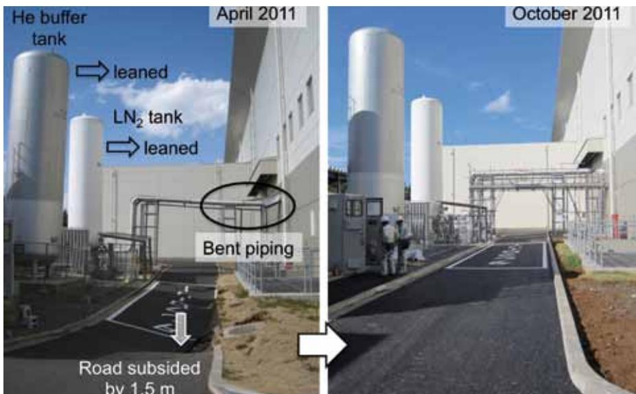
Figure 1: The liquid nitrogen storage tank and the helium buffer tank for the cryogenic hydrogen system leaned due to the ground subsidence (left), and uprighted (right). Picture courtesy of J-PARC
