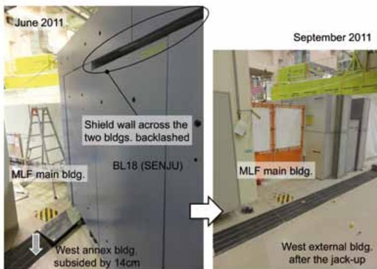
Figure 2: The subsided annex building (left) and that after the jack-up (right). Picture courtesy of J-PARC
